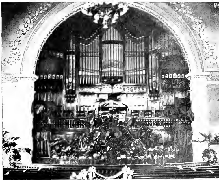
INTERIOR OF METHODIST CHURCH.
